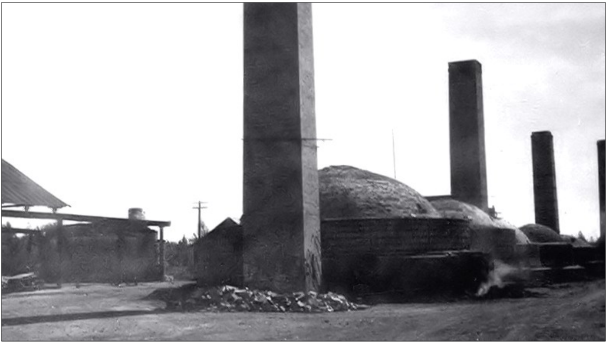
The west end of Washington Brick, Lime & Manufacturing Company's Clayton Factory — circa 1950. A portion of the framework for the plant's open kiln with sliding roof can be seen to the left side of the photo.
