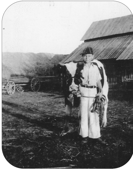
Wey at around age 10. The original barn is in the background. After the barn's hay storage area — the center area — had been filled, any extra hay was stacked outside (as seen near the corner of the barn in this photo). Being exposed to the ongoing effects of weather, this outside hay was always fed first. The milking area is the lean-to part of the barn.
