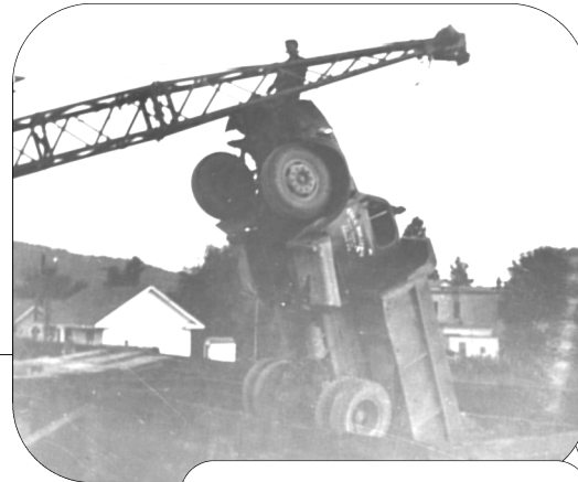
Above; the Richmond crane — near the loading ramp — removing the truck. Left; the truck sitting in the gondola.
