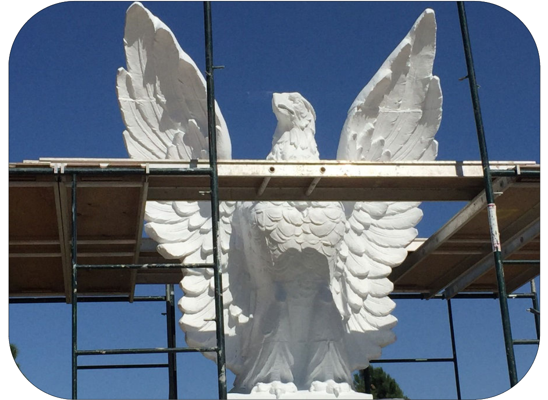
The thin membrane of “breathable” polyurethane sprayed on the sculpture acts to separate the aging terracotta from the elements, while allowing full exposure to those same elements.
