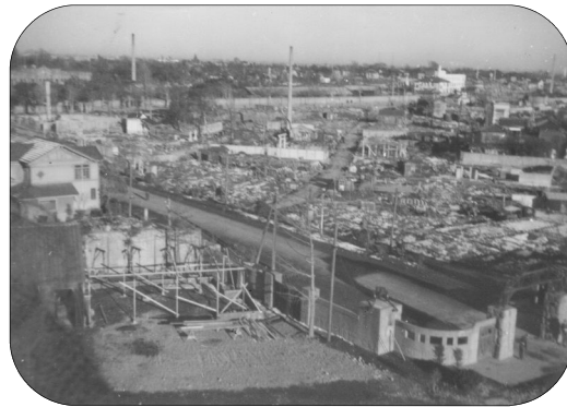
Viewed from the roof of the 8 th Cavalry building, you can see some of the damage to Tokyo and the random way in which damage occurred.
