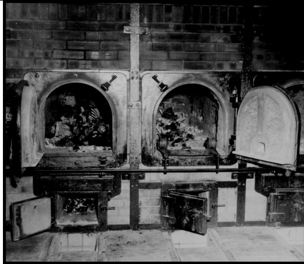
The furnaces at Buchenwald. Photo from the National Archives and Records Administration collection.
