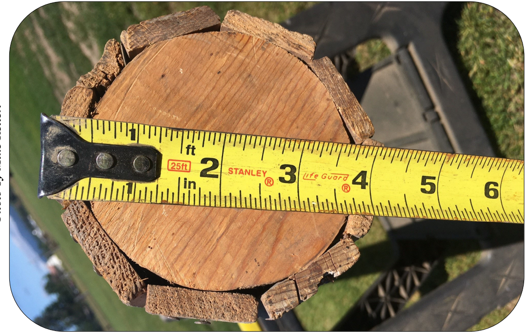
The Olsen Opera House's Olio Drop Curtain Roller. End view of the roller showing both the size and method of construction.
