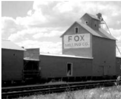
Photograph 2. Laswell Grain/Fox Milling warehouse and grain elevator in June of 1971.
