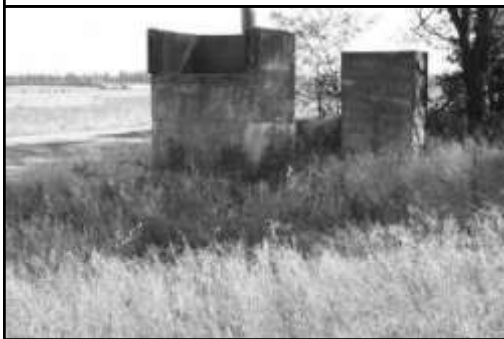
Photograph 4. Square concrete underpass flume supports on Antler road east of Cedar Road. Note the wooden blocks on the edges of the wooden flume support.
