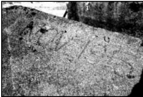
Photograph 8. "NOV 1913" scratched into the top of the Dragoon Creek dam.
