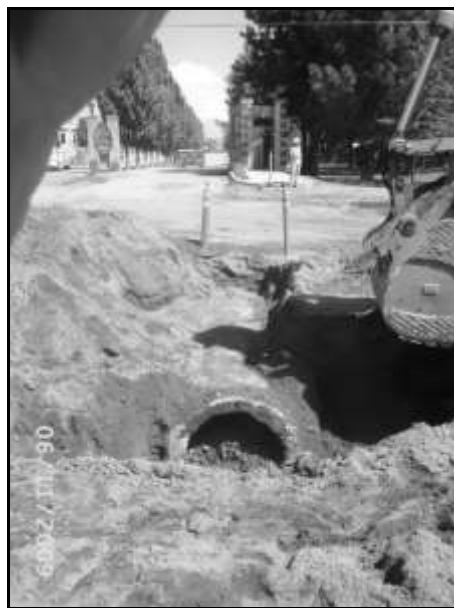
Photograph 5. Digging out the remains of a buried irrigation pipe on the east Crawford construction. (Photograph courtesy of the City of Deer Park and JUB Engineering.)
