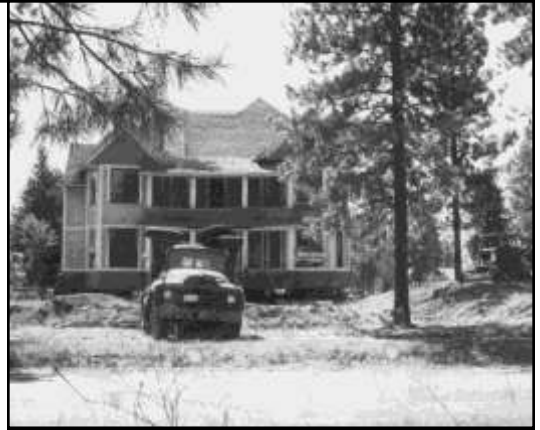
Photograph 7: The Kelly house being eased onto its new home. (Stephen Parkin Photograph)
