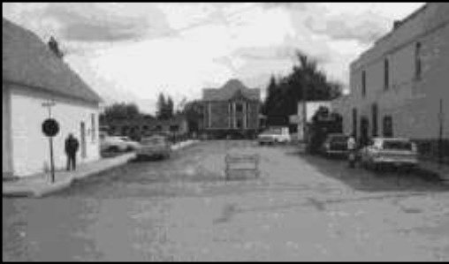
Photograph 5: East on First Street as the Kelly house is moved through the Vernon Avenue intersection. (Stephen Parkin Photograph)
