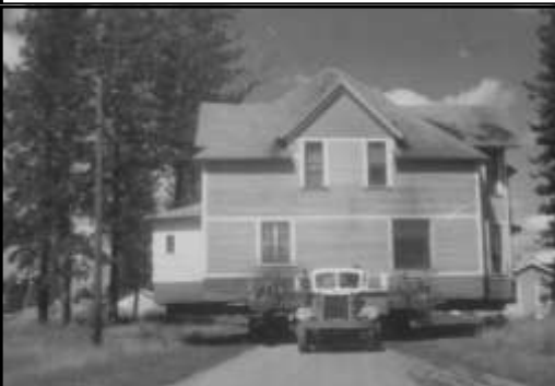
Photograph 6: The Kelly house moving slowly south on Vernon Avenue west of the swimming pool. (Stephen Parkin Photograph)
