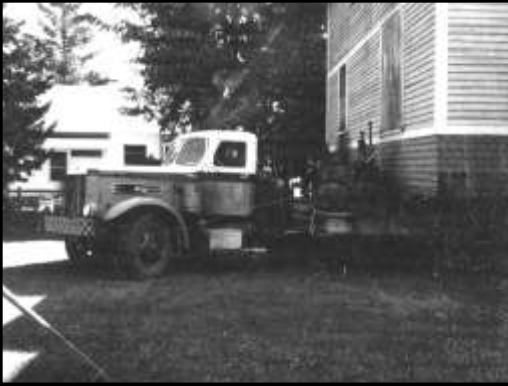
Photograph 4: The north side of the Kelly house on the moving truck as it begins its journey to the new location. (Stephen Parkin Photograph)
