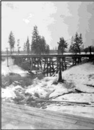
Figure 9: The Spokane Falls and Northern Railroad's trestle on Dragoon Creek just below the dam. A portion of the dam's wooden flood spillway is seen in the foreground. (Courtesy of the Northwest Room, Spokane Public Library)
