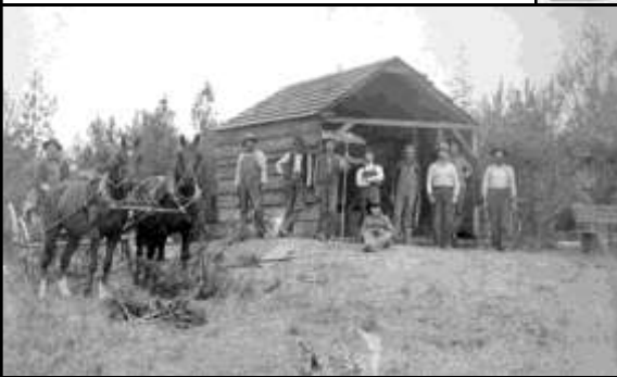
Figure 8: (Above) Photograph of a portable blacksmith shop used for equipment maintenance during the construction of the Arcadia Orchard canal system. (Courtesy of the Northwest Room, Spokane Public Library)
