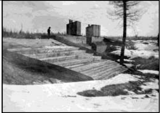
Figure 14: The finished Dragoon Creek dam with the flood spillway in the foreground with the dam and valve works behind it. (Courtesy of the Northwest Room, Spokane Public Library)
