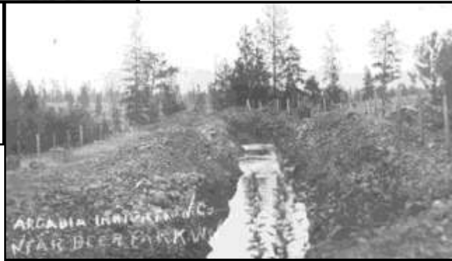
Figure 5: (Below) A water filled ditch cut into difficult ground near Deer Park. (Courtesy of the Northwest Room, Spokane Public Library)
