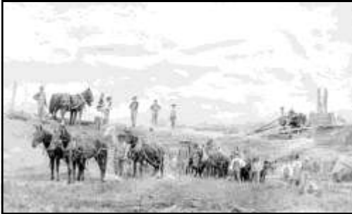
Figures 12 and 13: Photographs of the Dragoon Creek dam and spillway under construction. In the top picture the town of Deer Park can be seen in the background. The dam structure proper is the horizontally timbered structure in the center of the photograph. The function the steam tractor and the drive belt had is not clearly shown. (Courtesy of the Northwest Room, Spokane Public Library)
