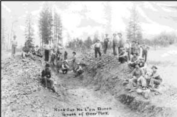
Figure 4: (Above) Ditch building south of Deer Park. This cut was most likely in the area of Dalton Road and US Highway 395. (Courtesy of the Northwest Room, Spokane Public Library)
