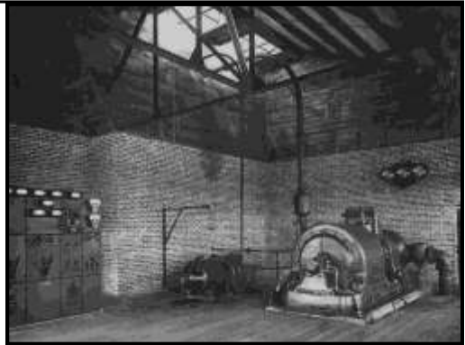
Figure 10: The General Electric Turbine on the left and the electric control panel on the right. Note the clean well kept appearance of the room and the brick walls. (Photograph courtesy of the Deer Park Open Door Congregational Church)
