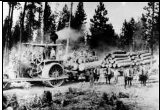
Figure 5: "Old Buck," the steam traction engine and loaded wagons on a dry road. The horse teams would skid the logs to a landing where they could be loaded on the wagons. (Photograph from the Lawrence Zimmerer Collection)
