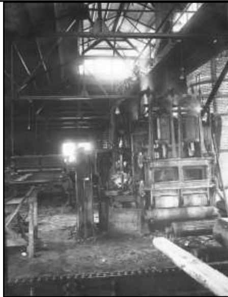
Figure 8: The Diamond edger is on the left and the gang saw is on the right. In the right foreground a rough board and a cant are on the chain coming from the band saw. (Photograph courtesy of the Deer Park Open Door Congregational Church)
