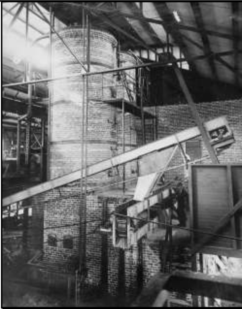
Figure 9: The cylindrical brick Wickes Brothers' boilers behind the scrap conveyor in the foreground feeding the furnace. (Photograph courtesy of the Deer Park Open Door Congregational Church)
