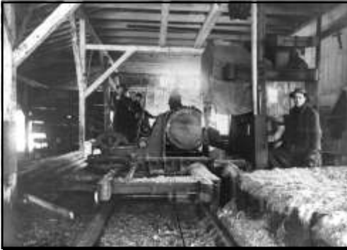
Figure 4: Inside the first Standard Lumber Mill Company's mill. Note that the mill is composed of two large circular saw blades set one above the other. The sawyer stands to the right and the setter rides the carriage back and forth in front of the saws. The building is constructed of wooden timbers.
