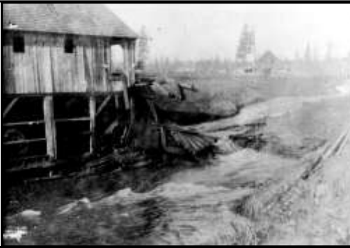
Figure 2: The upstream corner of the Gemmill Mill and the flood damage that washed away the flume. Dragoon Creek still looks to be in flood! (Photograph from the Lawrence Zimmerer Collection)
