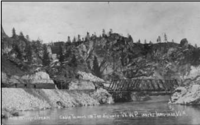
Figure 4: The southern terminus of the Springdale and Long Lake Railroad during construction of the dam with a bridge across the Spokane River. The Long Lake Dam site is just to the right of the picture. (M. Denuty postcard collection)
