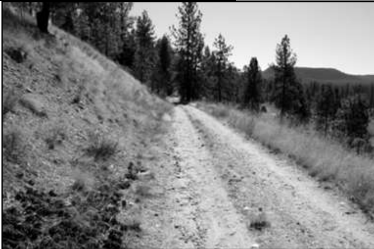
Figure 3: South along the remaining Springdale and Long Lake Railroad right of way cut into the steep slopes just north of the Spokane River. The road bed is used as an access road to power lines which take electricity north from the Long Lake Dam. (Coffin Photograph September 2010)
