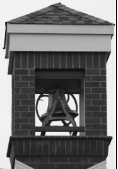
Right: Figure 5: Deer Park Elementary bell tower from the southwest. Note the slack piece of cable on the upper left of the ringing wheel. (P. Coffin Photograph, March 20, 2011)
