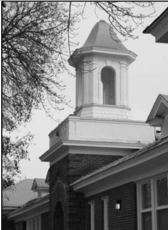
Figure 1: The Deer Park School Administration Building bell tower from the southwest on March 20, 2011. The tower is empty! (P. Coffin Photograph)
