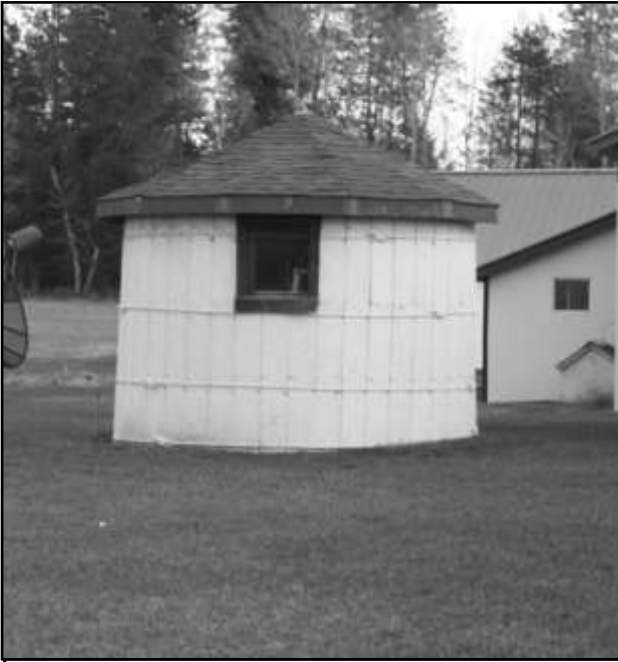
Figure 3: The roof of the concrete stave silo at Whittier and Cowan Roads. (2011 P. Coffin Photograph
