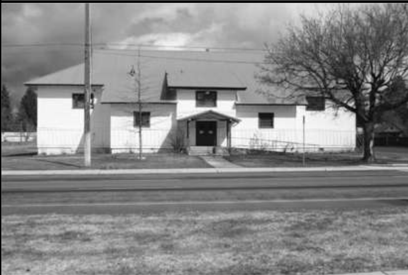
Figure 8: The first Deer Park Gymnasium as the Deer Park Community Center in April 2011. The building appears as it did when built! (Peter Coffin Photograph)
