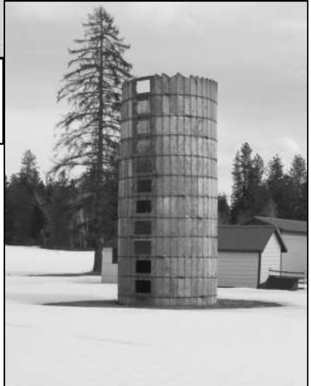
Above: Figure 1: Concrete Stave Silo at Whittier and Cowan Roads from the south. (2011 P. Coffin Photograph)
