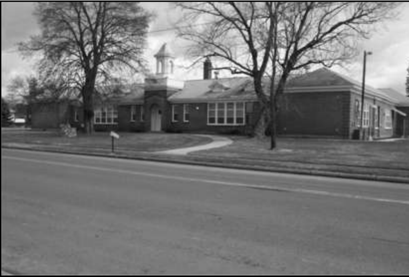
Figure 7: The 1922 grade school as it appears in April 2011 as the School Administration Building. From the front the building appears as it did when built. (Peter Coffin Photograph)
