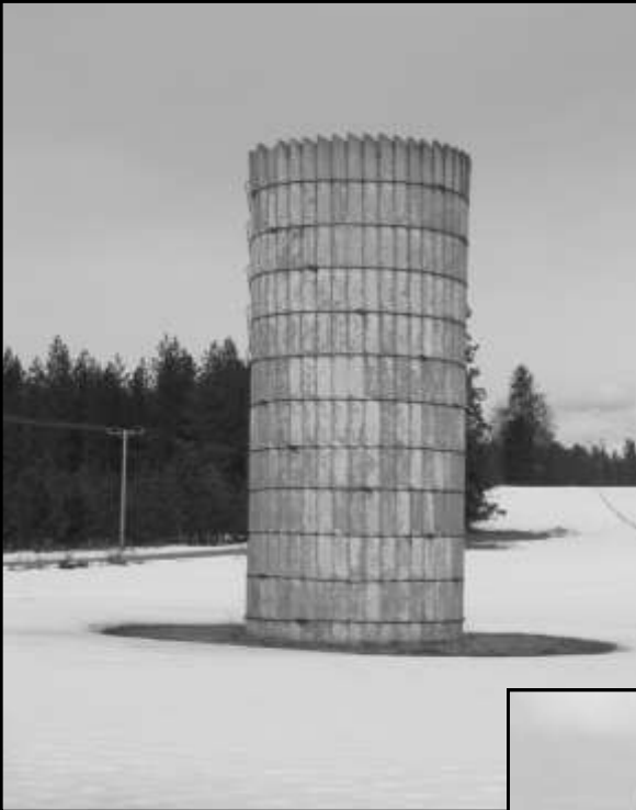
Above: Figure 1: Concrete Stave Silo at Whittier and Cowan Roads from the south. (2011 P. Coffin Photograph)
