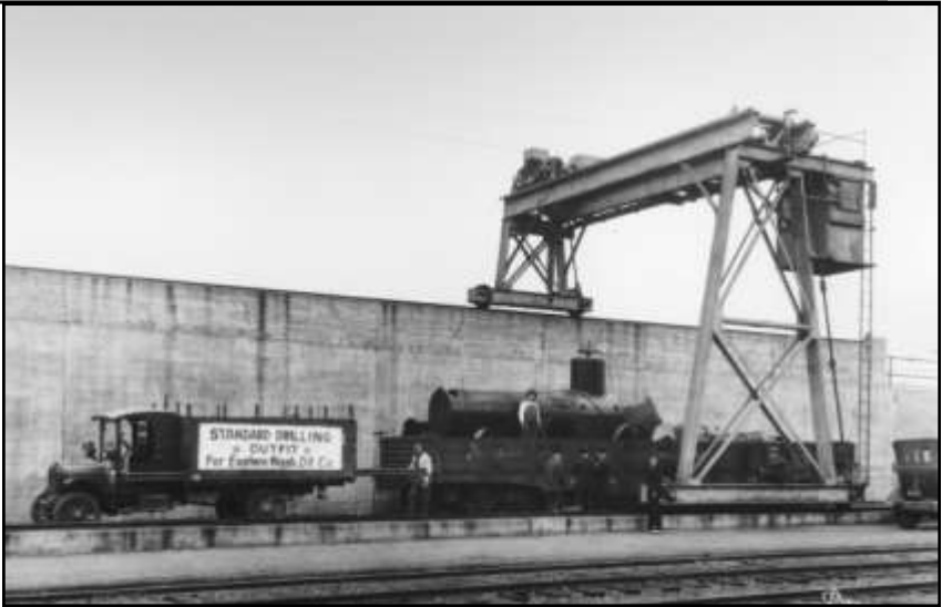
Figure 2: Photograph of parts of a “Standard Drilling” rig being delivered to Spokane and the Eastern Washington Oil Company for use in the 1921 drilling boom. The boiler would have been used to generate steam for the cable tool drilling machinery.
