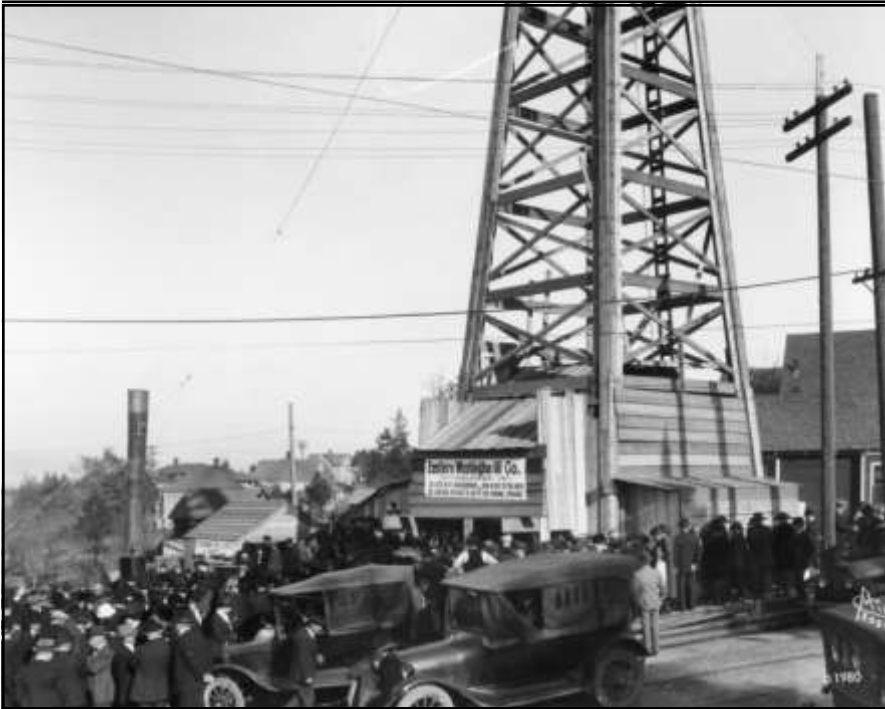
Figure 4: Photograph of one of the derricks drilling for oil on Spokane's south hill in 1921. Location is shown on the map in Figure 3. This type of timber derrick would have been used for drilling in the Deer Park and Clayton area. (Photograph from the Collection of Gerald Quinn)
