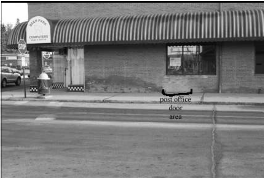
Figure 3: The west side of the hotel shows the bottom outline of the door that led to the post office (P. Coffin Photograph January 2012)
