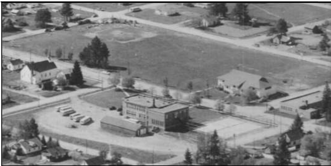
Figure 2: Aerial view of Deer Park High School showing the 1936 addition as it comes off the east and southeast sides of the building. Scamahorn Photo circa 1953.
