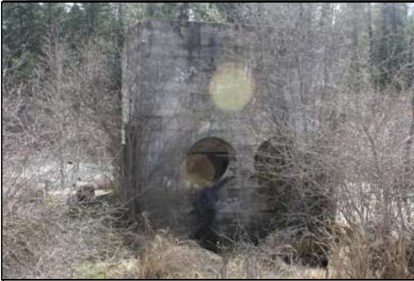
Figure 5: Holes in the north side of the “generator house” to receive the water from the weir/dam. (March 2013 Coffin photograph)
