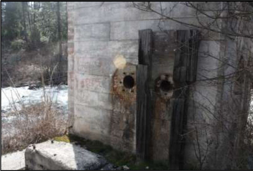
Figure 7: Holes on the east side of the “Generating House” that may have supplied water to a generator inside the brick building seen in early pictures of the site. (March 2013 Coffin photograph)
