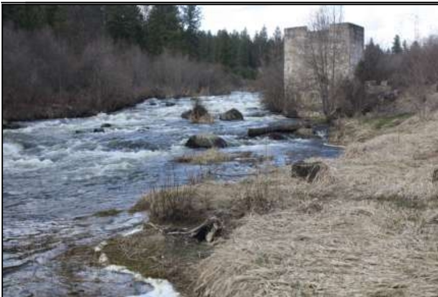
Figure 3: The concrete tower remaining next to the Little Spokane River. Early pictures show water spilling over the notch in the top of the tower. (March 2013 Coffin picture)
