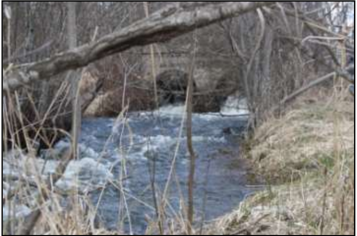
Figure 4: Downstream view of the weir/dam with the large cast holes for the pipes to carry water to the generators. The weir has been broken and water is flowing through both the holes and the eastern side of the retaining walls. )
