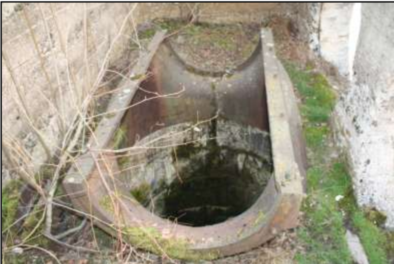
Figure 6: Rusting iron frame inside the “generator house” that may be a turbine base. To the right are the large circular holes that conducted water into the structure. (March 2013 Coffin/Luiten photograph)
