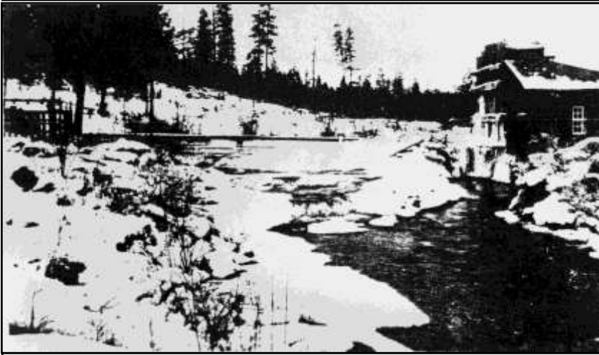
Figure 2: View of the Little Spokane Power plant and what appears to be a dam in the left center of the picture. Today nothing remains of this structure (Photograph from the Lawrence Zimmerer Collection)
