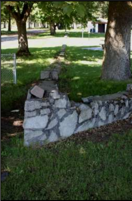
Figure 4: Masonry wall at the southeast corner of the original city park. The Tourist Park “motel” used to be located in the area of the upper left corner of this photograph. (P. Coffin, 2013 photograph).
